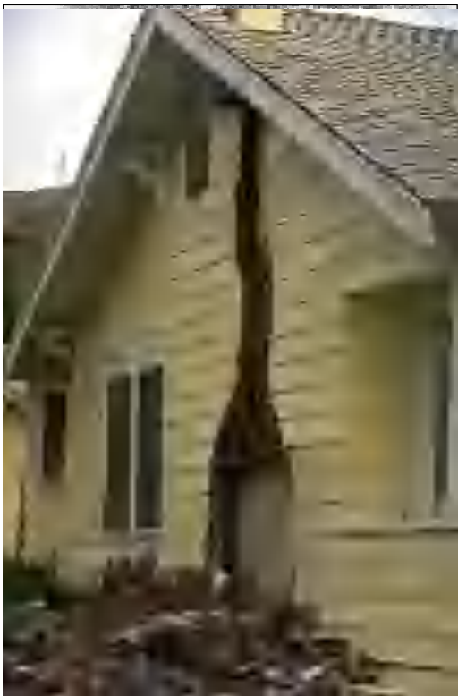
Chimney collapse is a widespread problem.
