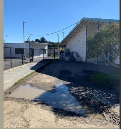
Asphalt paving adjacent to Annex building is in need of repair and selected replacement. Annex building should be demolished.
