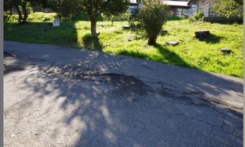
Parking lot paving outside of preschool requires repair, infill of potholes and repaving.
